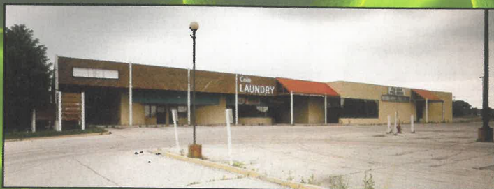
Washington Square Mall was abandoned after a toxic chemical known as PCE leaked into the groundwater.
